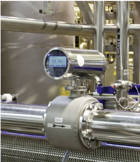
Flow measurement in flash pasteurizer
